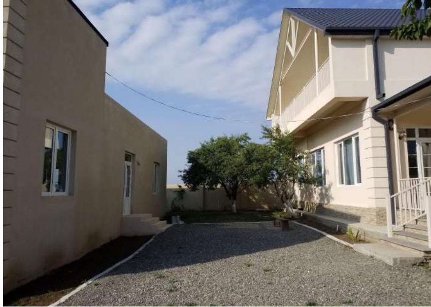
ECG's first and second buildings are on the same land plot; the distance between them is six meters (19.5 feet), 2022
