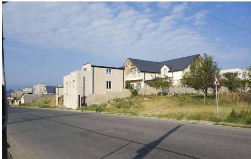
The exterior of the completed ECG prayer house, both buildings, 2022
