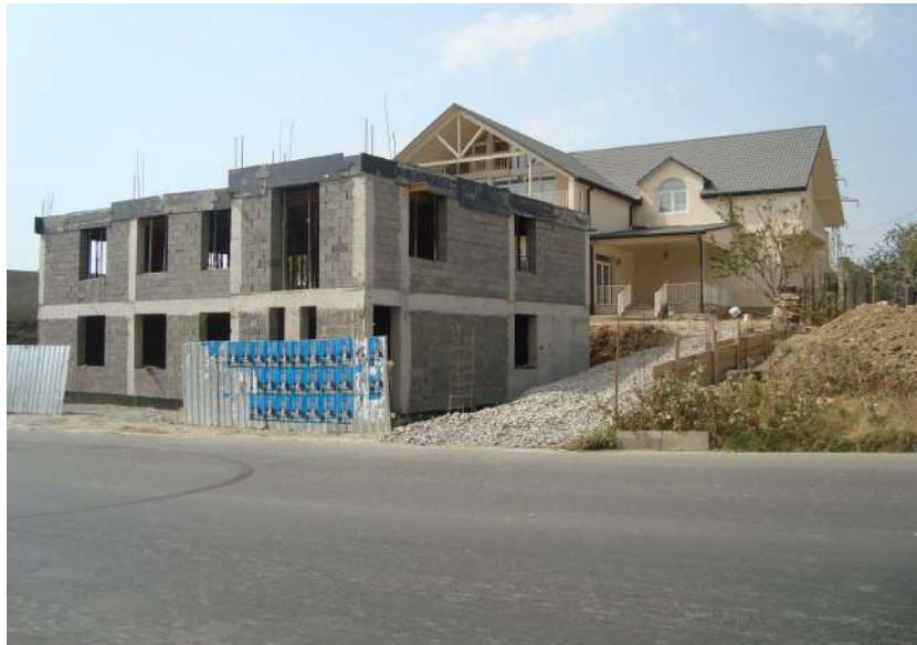
The construction process of ECG's second building, 2017
